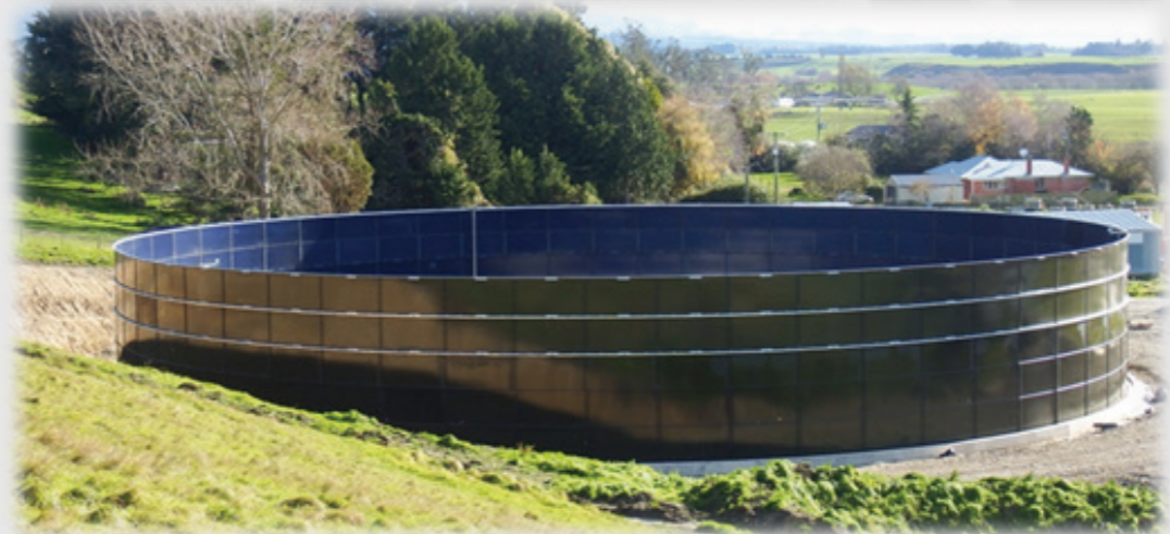
Bulk water storage
